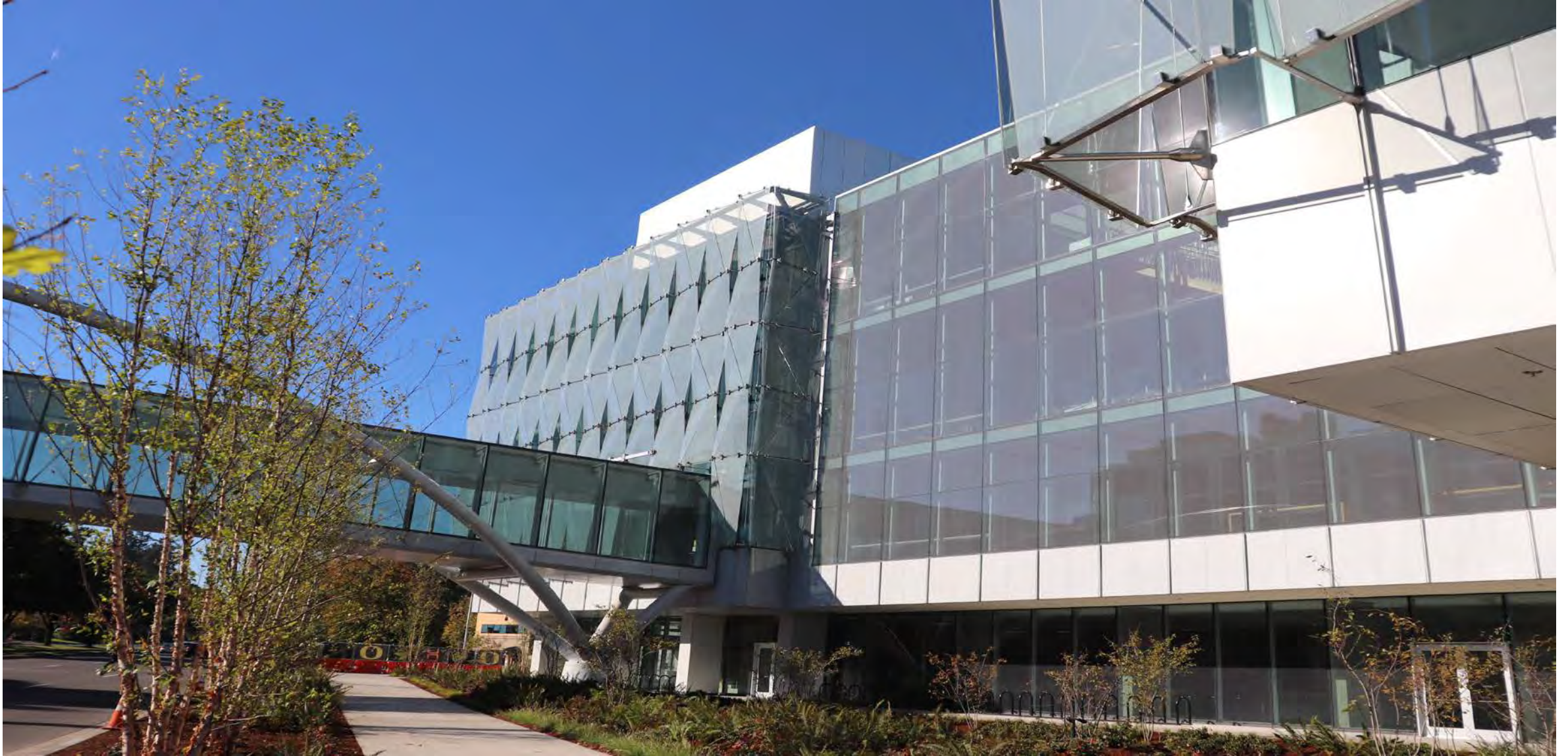
Front of the building looking at “the connector,” the West Tower, and the bridge connecting the Knight Campus to the Lewis Integrated Science Building on the main UO campus.
