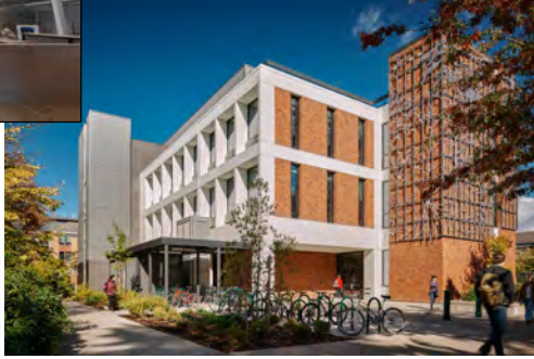
Huestis Deferred Maintenance – Recently Completed (photo: @Ryan Gobuty)
