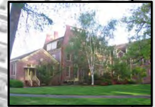
Hendricks Hall Deferred Maint.
