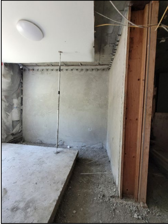
New shear wall located in a student room
