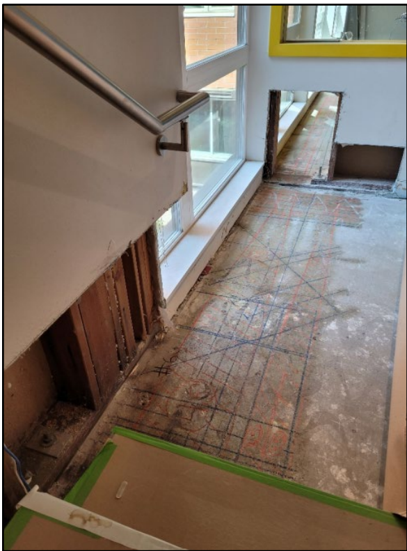
Ground penetrating radar scanning lines of tie strap plates
