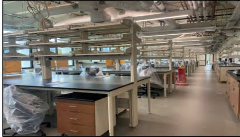
Huestis Deferred Maintenance – In Construction
