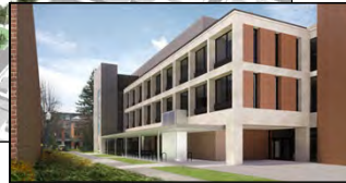
Huestis Hall Deferred Maintenance
