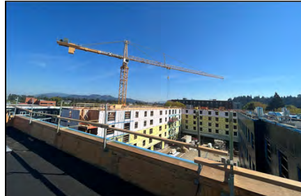
Housing Transformation Project: Phase 2 (Walton) – Under Construction
