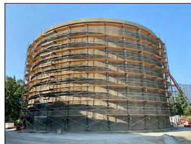
Chilled Water Tank – Under Construction
