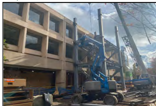
Huestis DM– Under Construction
