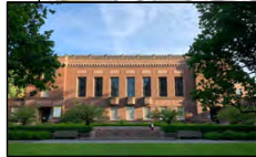
Knight Library Exterior Restoration
