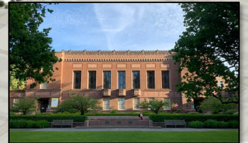
Knight Library Exterior Restoration
