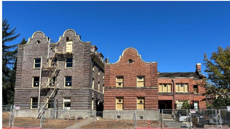
Friendly Hall – In Construction
