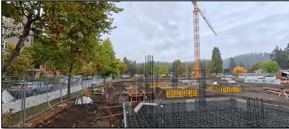
Housing Next Generation Building 1 – In Construction
