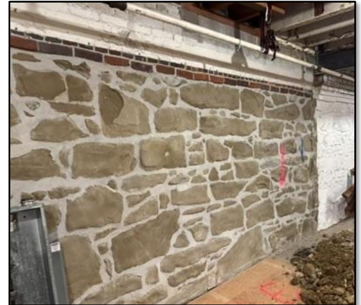
Example of an unreinforced masonry foundation. Friendly Hall - currently under rehabilitation.
