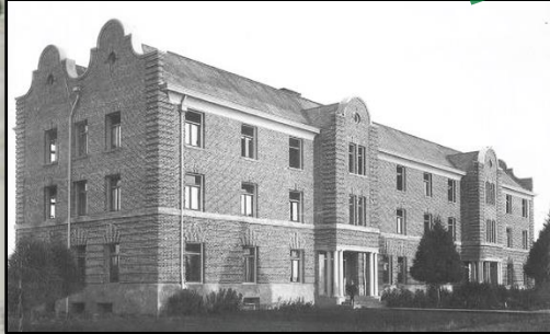
Friendly Hall Deferred Maintenance
