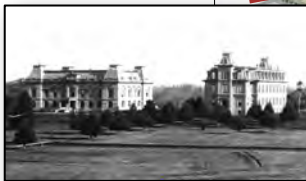
Heritage Project: University and Villard Hall Deferred Maintenance
